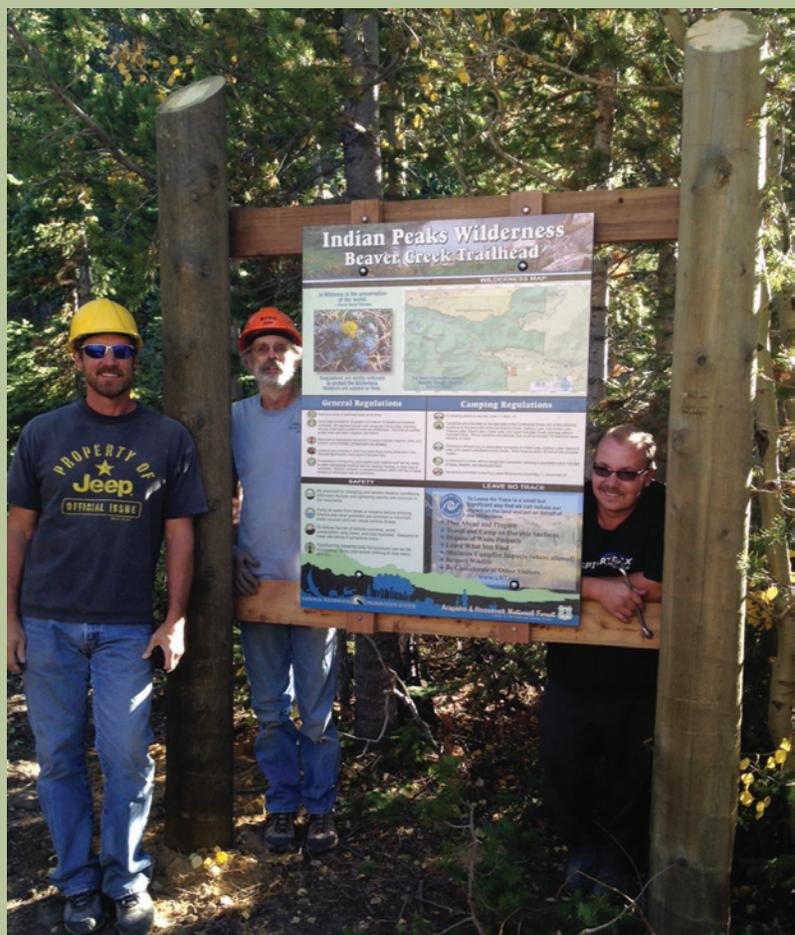
We got the support post cut to length and placed in the holes while the sign cross supports were getting laid out and pre-drilled. Once all the pieces were ready the cross supports were installed and then the new trailhead sign was bolted on.
